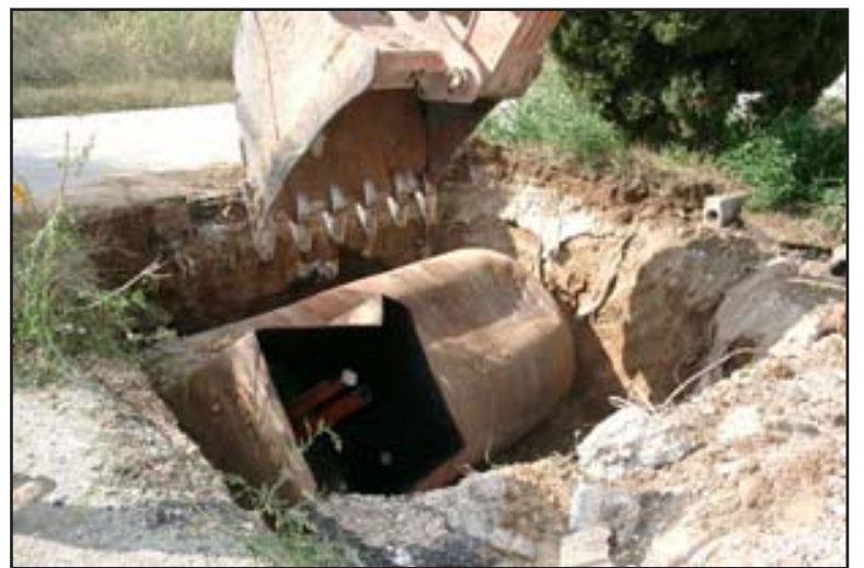
A backhoe prepares to remove an underground storage tank from Dal Molin. (Photo courtesy of the Transformation Construction Management Office)
